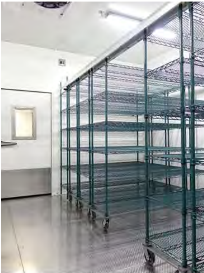
The Metro Top-Track, High-Density Storage System is a versatile storage system that allows maximum use of floor space. (Inside of the 30°C/65% RH walk-in chamber looking at the Metro Top-Track, High-Density Storage System.)
