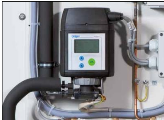
Figure 16: Fire Detection via CO Gas Monitoring
